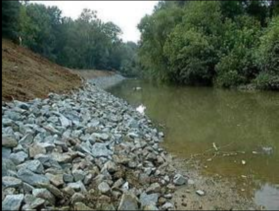
Stream Bank Erosion
