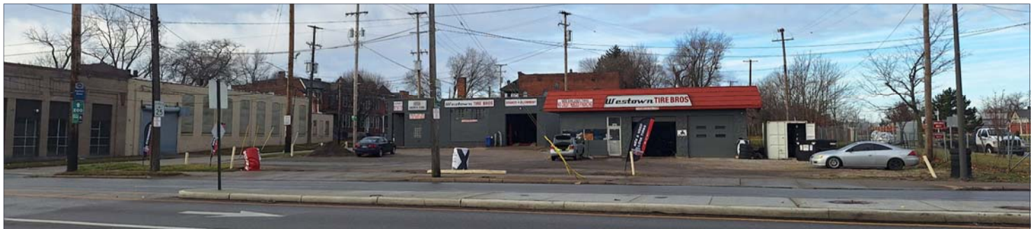
Existing site photo of Westown Tire
