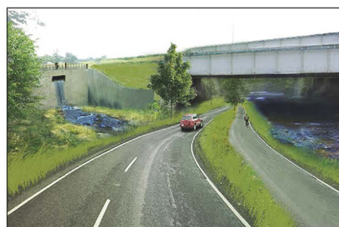
Big Creek in Cleveland Metroparks Brookside Reservation: existing drop structure (left) and proposed realignment (right)
