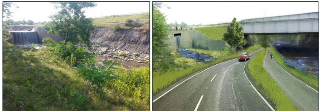
Big Creek in Cleveland Metroparks Brookside Reservation: existing drop structure (left) and proposed realignment (right)
